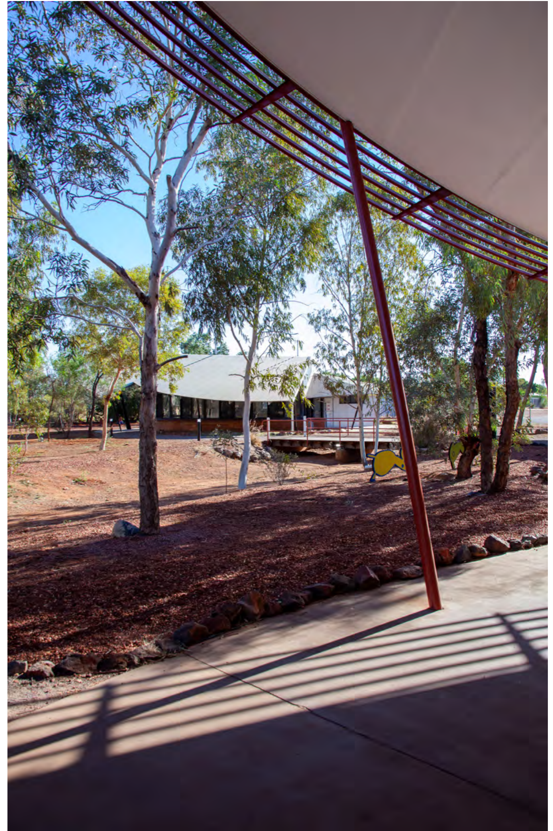
↑ Sweeping canopies create shaded spaces on the edge of the building and soften the space between the building and the bush garden. The iron red columns, both round and spliced, are intended to evoke tree trunks found across Warumungu Country.
