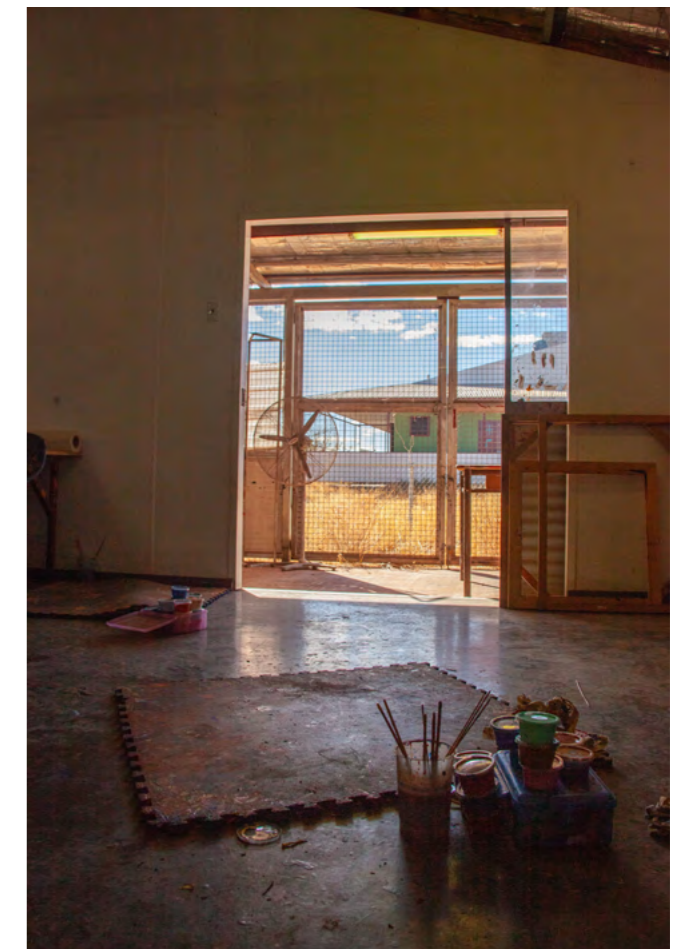
↑ The studios have access to semi-exterior spaces, however these areas are undersized and either poorly oriented toward the west or exposed to public areas. These openings are one of the only access points to natural daylight in both of the art studios. The existing sliding doors offer poor protection from dust and wind.
